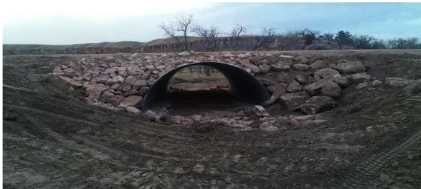
Figure 5. New Bridge over a Problematic Area
