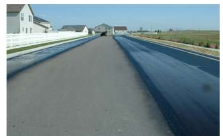
Figure 3. GSB-88® Applied on a Residential Street.
